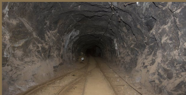
The Main Hereditary Adit below the power plant
